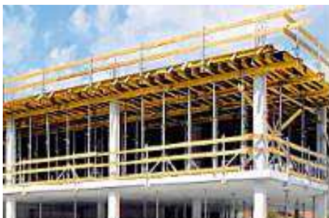
floor full concrete
