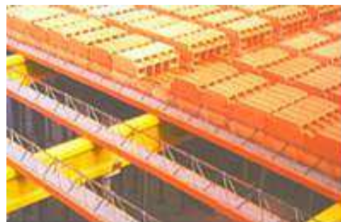
floor with precast beams
